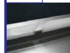
Allow a space of approximately 10mm between two slide rail ends.
