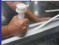
Use the slide rail assembly tool to press the slide rail into place.
