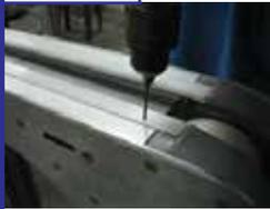
Drill two holes near the beginning of each slide rail section. Use the drill fixture to ensure clean-cut holes and correct location of the holes. The holes must be at the beginning edge of the joint piece, in the direction of travel, to hole the slide rail in place when the conveyor in use. Use a well-sharpened drill bit.
