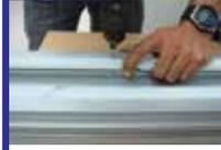
Drill through holes on slide rail.
