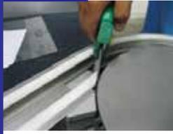
Cut the slide rail end in a 45° angle.
