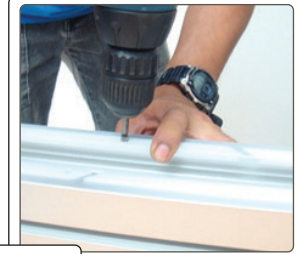
2 Countersink hole on slide rail.
