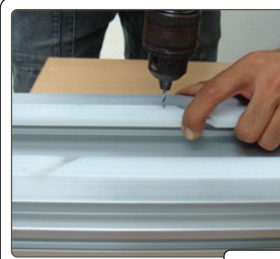
Drill through holes on slide rail.
