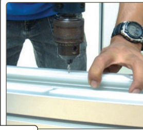
1 Drill through holes on slide rail.
